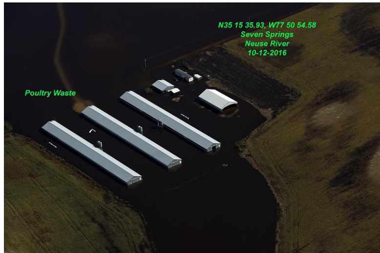
Figure 4 Poultry Waste Storage After Hurricane Matthew
