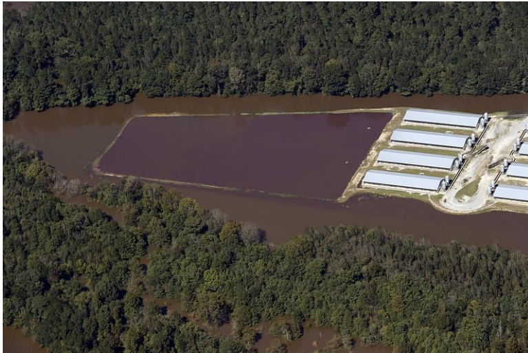
Figure 3 Hog Waste Lagoon After Hurricane Matthew
